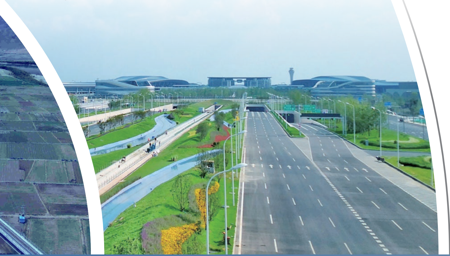
Tunnel underneath North Taxiway of Chengdu Tianfu International Airport
